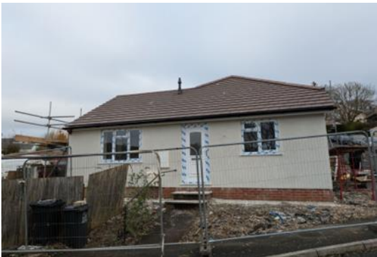
Fig. 2. Nearing completion of re-instatement.
